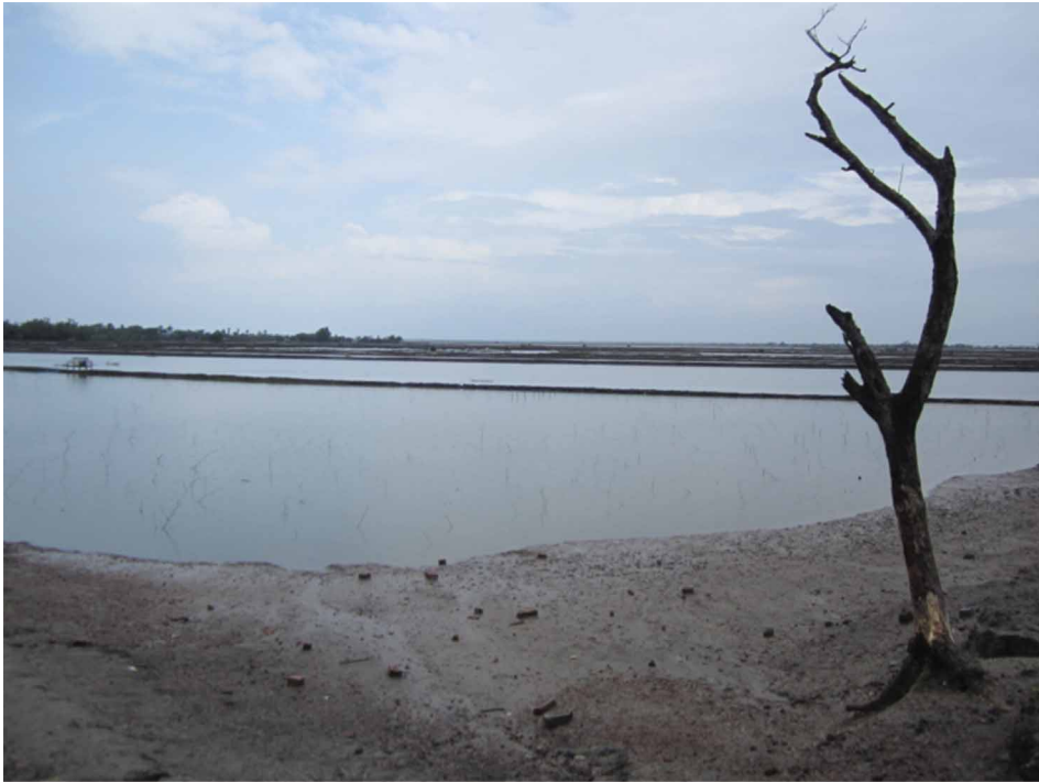
Figure 2. View from inside Polder 23.
